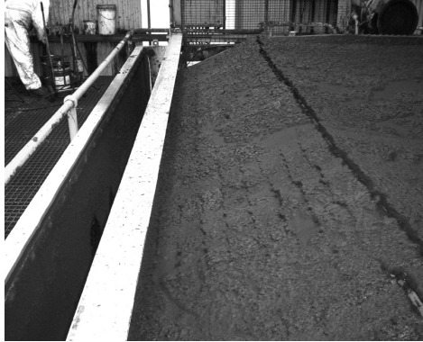
Figure 4 Discharge End of Conveyor Prior to Installation
