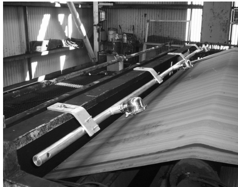
Figure 5 Installation of Sensor Heads During Shutdown Period
